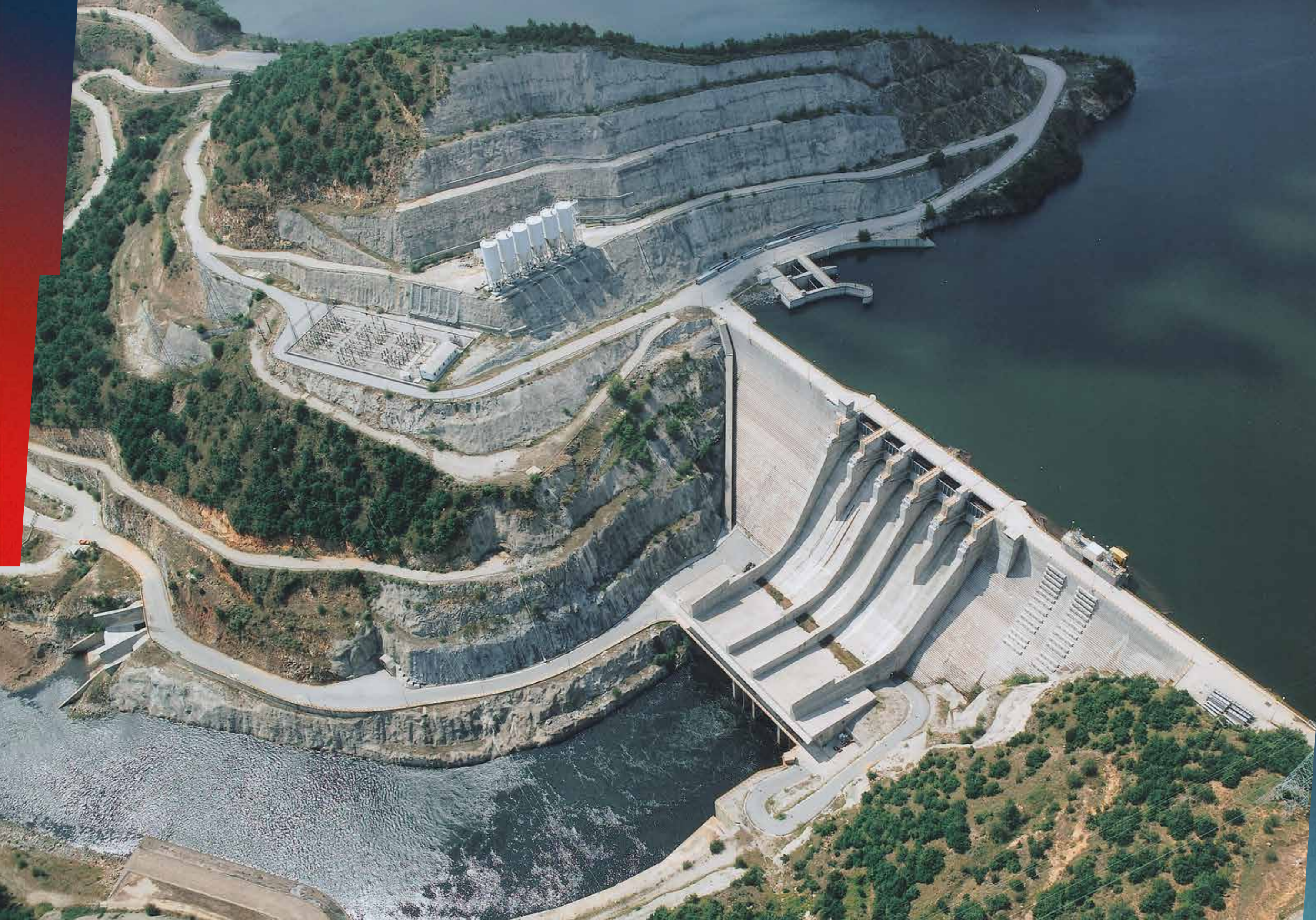
Hydroelectric Power Plant Dam - Platanovrshi
