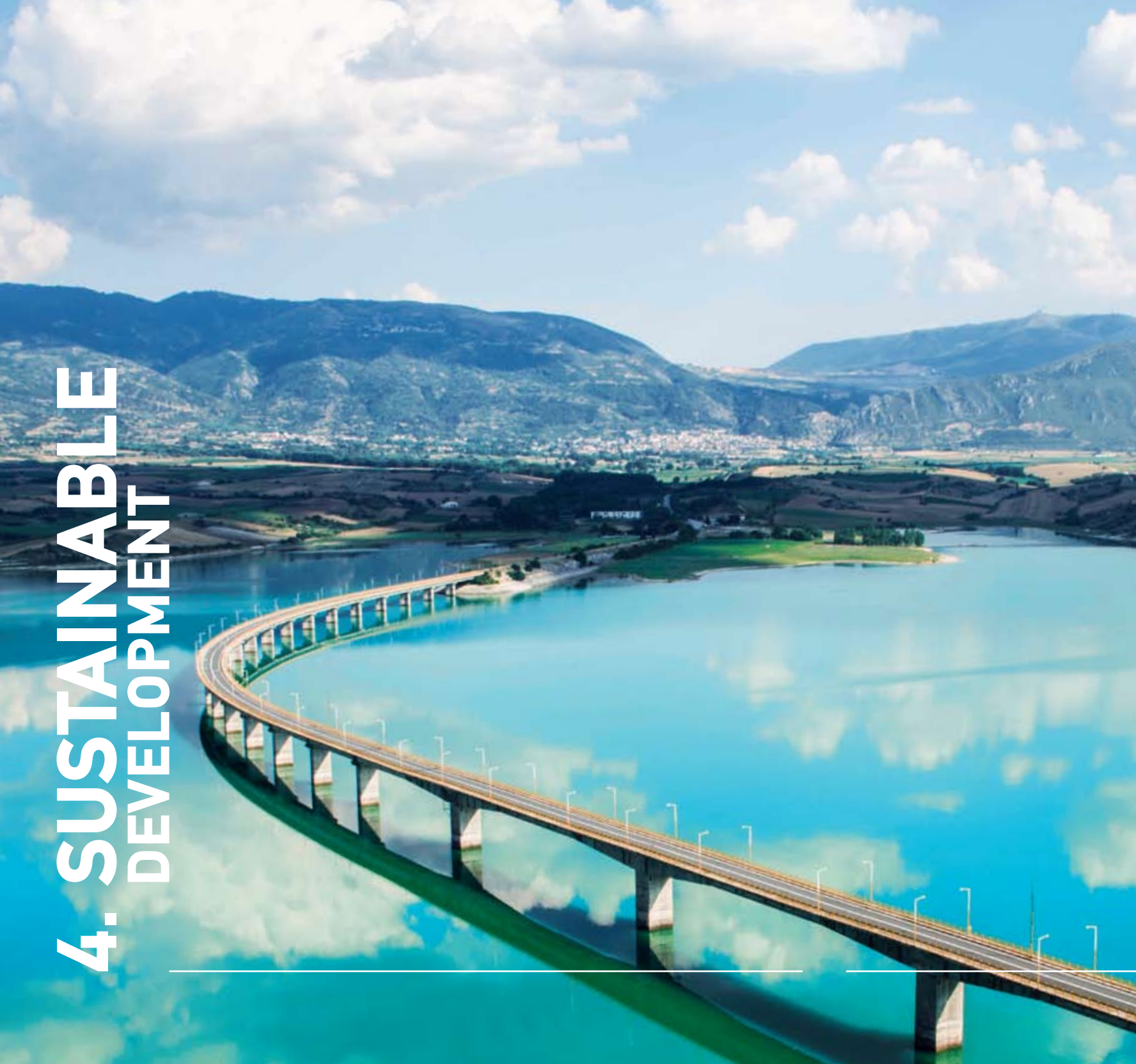
Servia High Bridge - Polyfyto Artificial Lake
