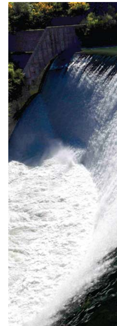
Louros HPP Dam
