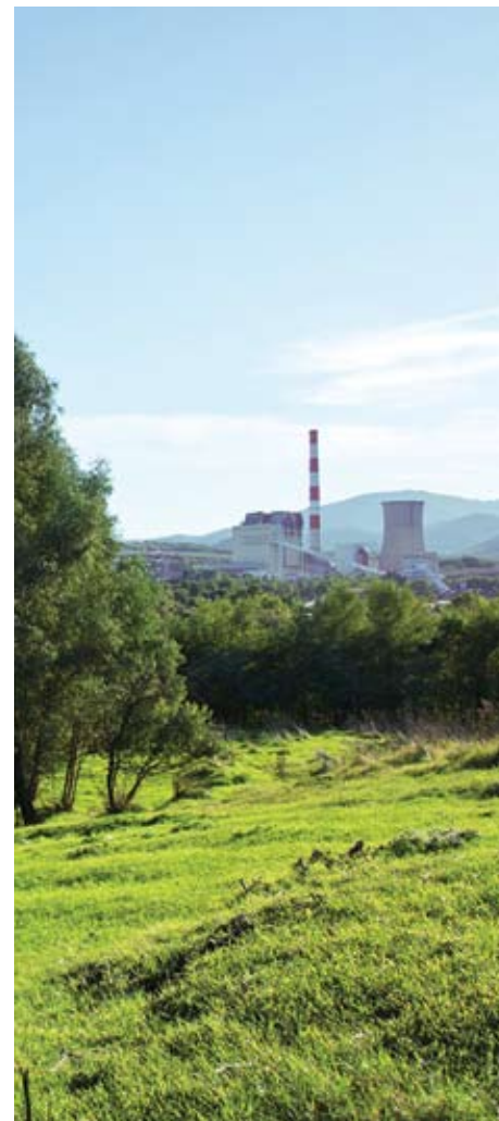
Rehabilitation of land, Megalopolis Unit IV
